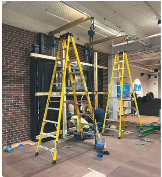
L to r, L-744 Boilermakers Heath Vincent and Greg Pame secure posts to the facade.
