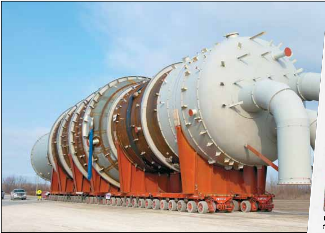
A VACUUM FLASHER TOWER weighing nearly 1,000 tons is moved toward the refinery after being offloaded from a Mississippi River barge.
