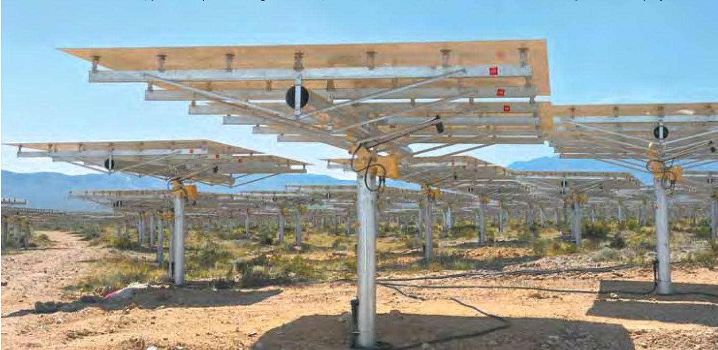
AN ARRAY OF MIRRORS , pointed skyward during installation, are a fraction of the 173,000 heliostats that will be placed on the project site.
