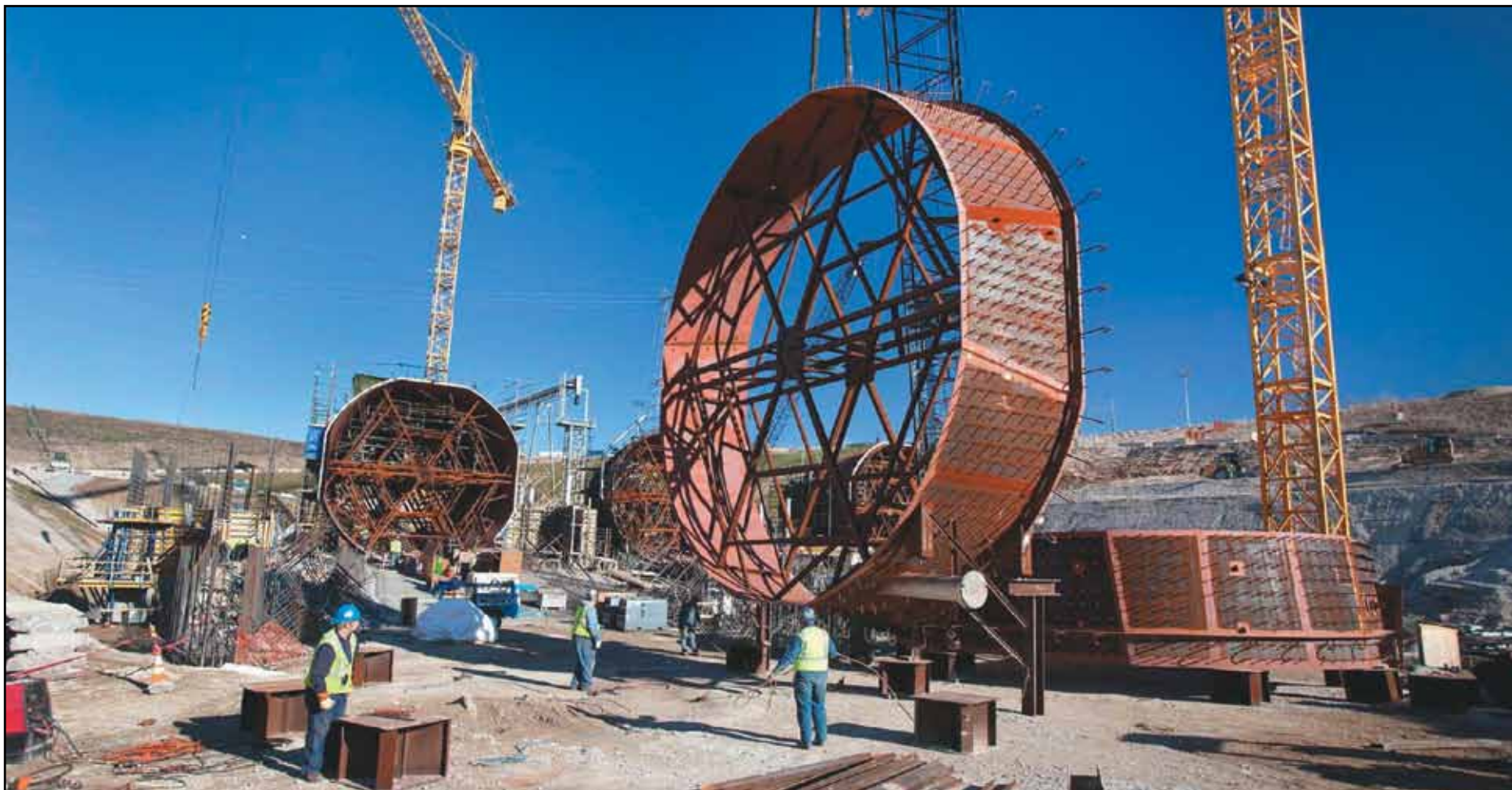
BOILERMAKERS MAKE A LIFT inside the 10-story cofferdam that parallels the river. All photos courtesy of National Steel Erection, Inc.
