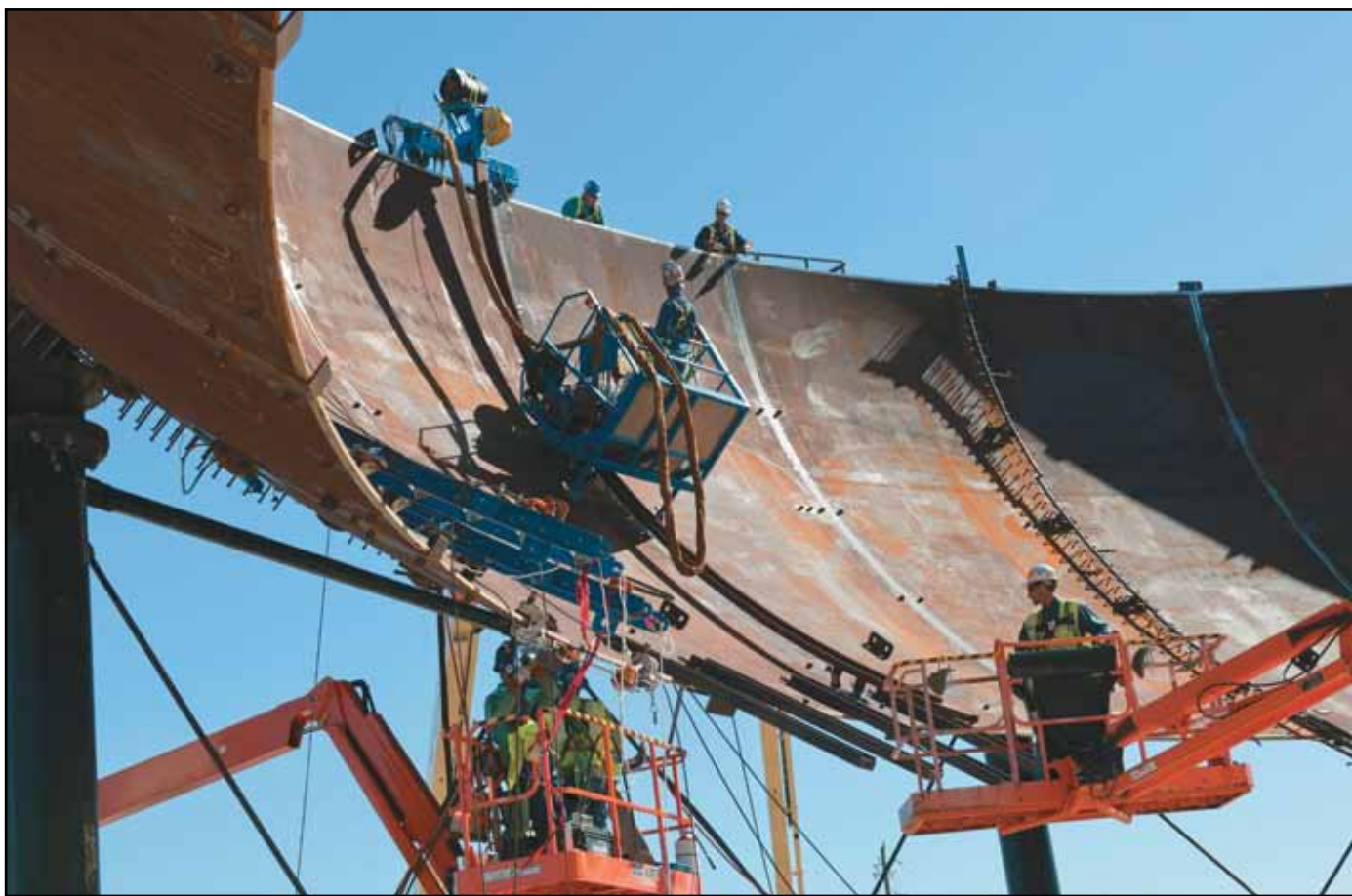
BOILERMAKERS WELD some of the 58 steel plates that will form the Vogtle unit 3 containment vessel bottom head. Courtesy Southern Company, all rights reserved
