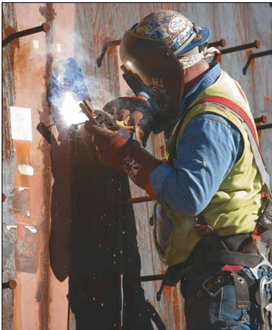
L-363 (EAST ST. LOUIS) MEMBER JEREMY DYE makes a weld on the outside of adjoining tube liner sections at the Cannelton hydroelectric power project.
