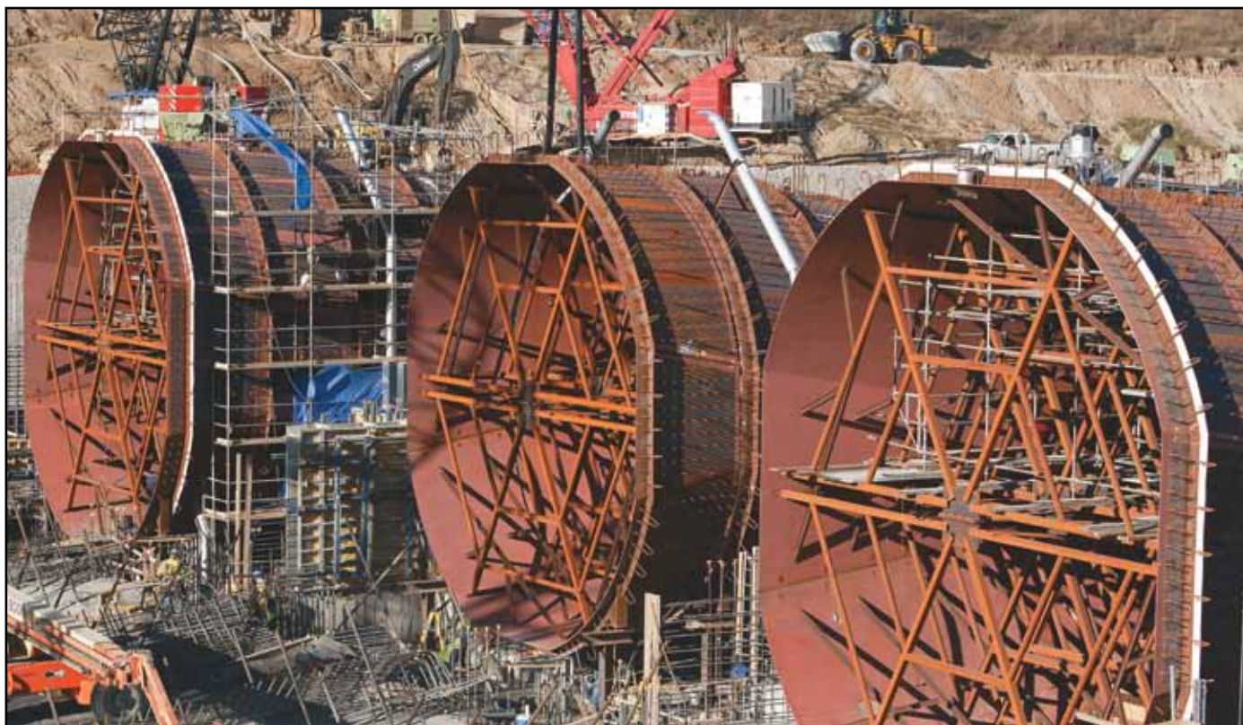
WATER FROM THE OHIO RIVER will rush into the hydro tube liners, turning the power plant's three turbines.
