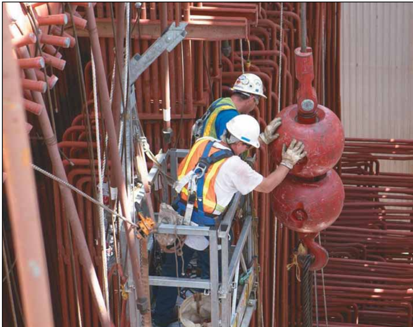
TWO BOILERMAKERS HELP DIRECT A TUBE SECTION LIFT. Photo courtesy of MOST/Martin Public Relations
