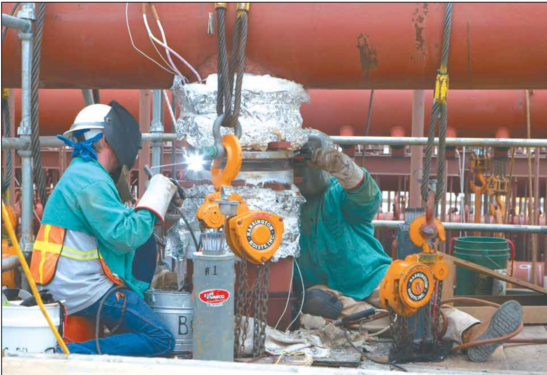
BOILERMAKERS perform one of the many high-pressure, heavy-wall boiler welds at the Turk project.
