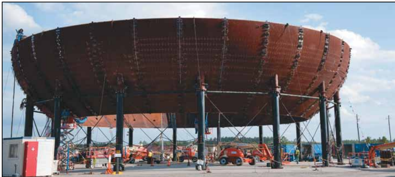
UPPER SECTION OF VOGTLE UNIT 3 containment vessel lower head, fastened to assembly and welding stand. Courtesy Southern Company, all rights reserved
