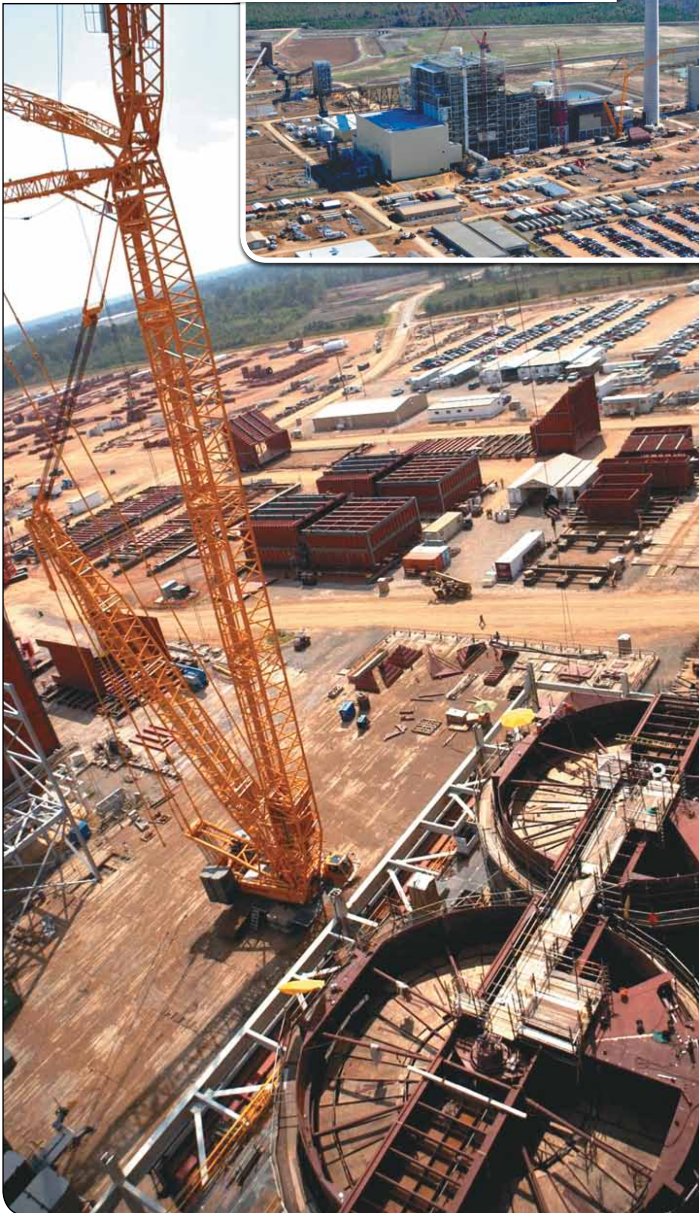
AIR HEATERS are pictured in the foreground. At top is the extensive lay-down yard.
