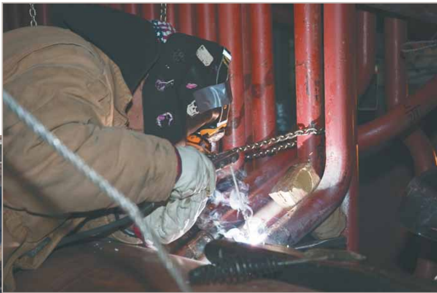
MARCO MARTINEZ, L-5 , performs a weld on a unit 2 economizer header. Welding partner Tim Booth, L-363 (off camera) welds on the opposite side of the tube.
