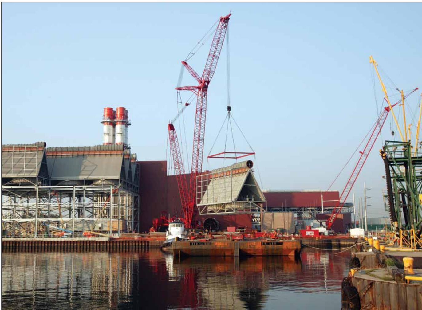
A MODULE IS LIFTED from a barge before being placed atop support structure at the Astoria Energy project in New York City.
