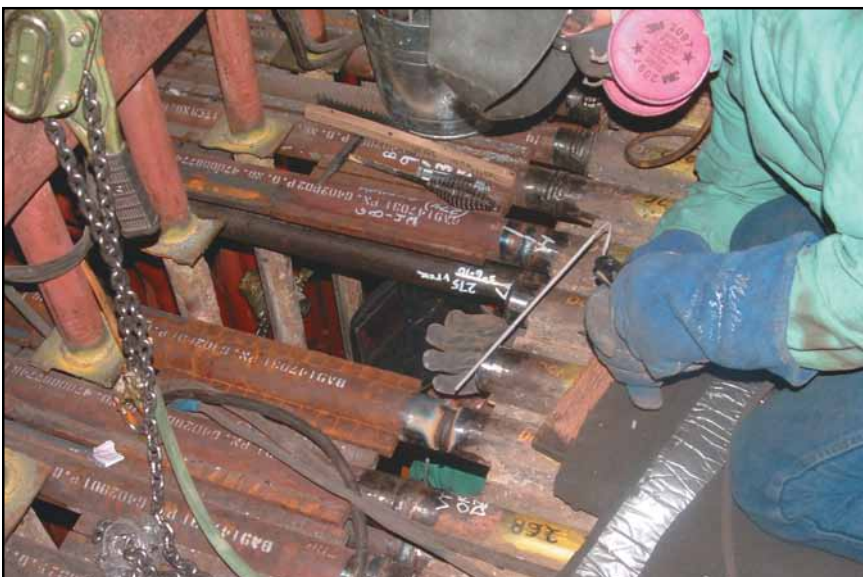
LOCAL 85 MEMBERS JOEL CLARK and Abe Babcock make a roof tube weld. Babcock is under the structure; only his glove and welding shield are visible.
