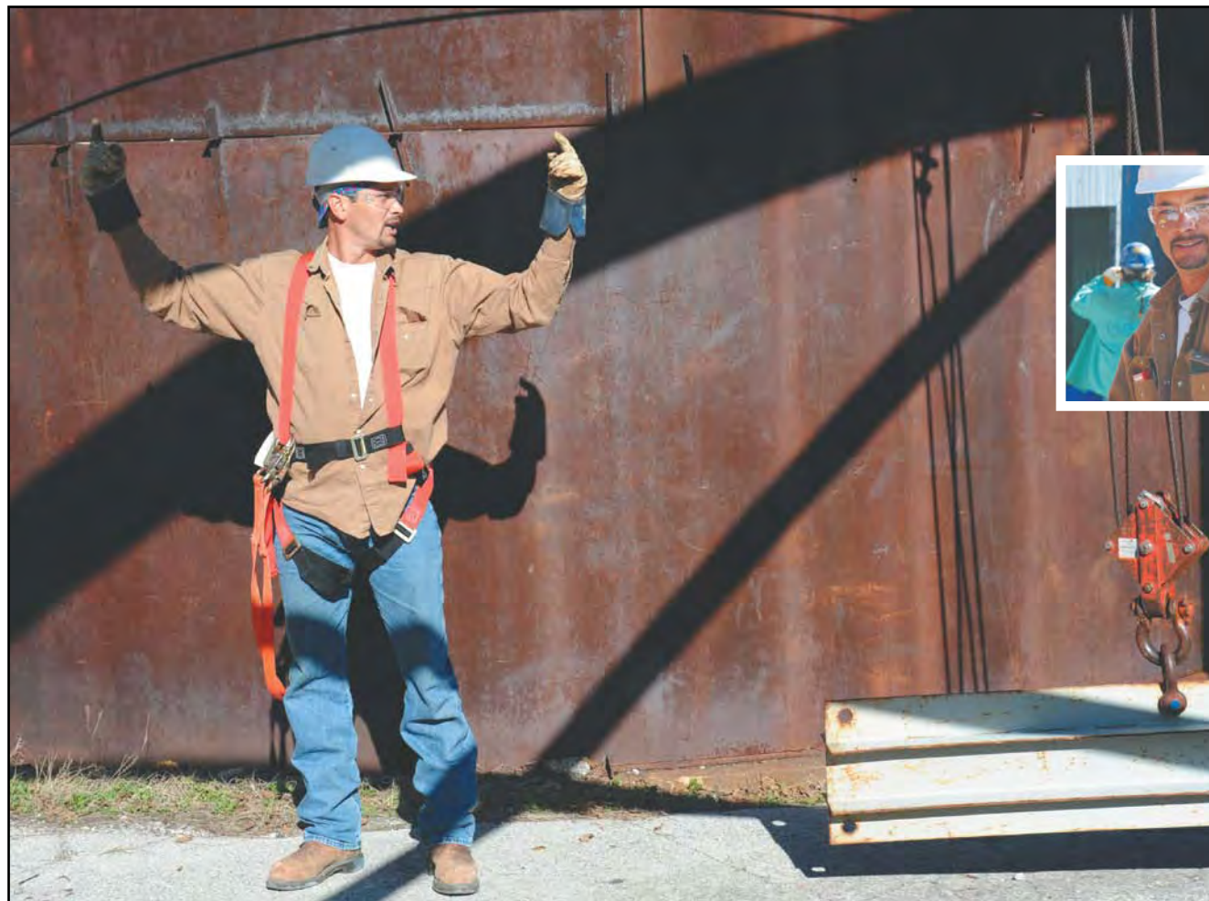
Thomas Tucker, Local 69, shows his dual flagging skills to position an equalizer beam.
