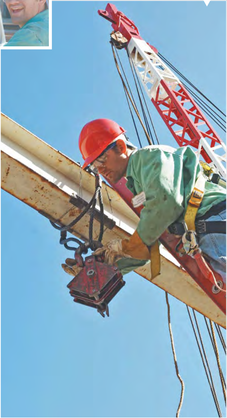
Matthew Vodraska, Local 744, hangs a block from a beam during the rigging exercise.
