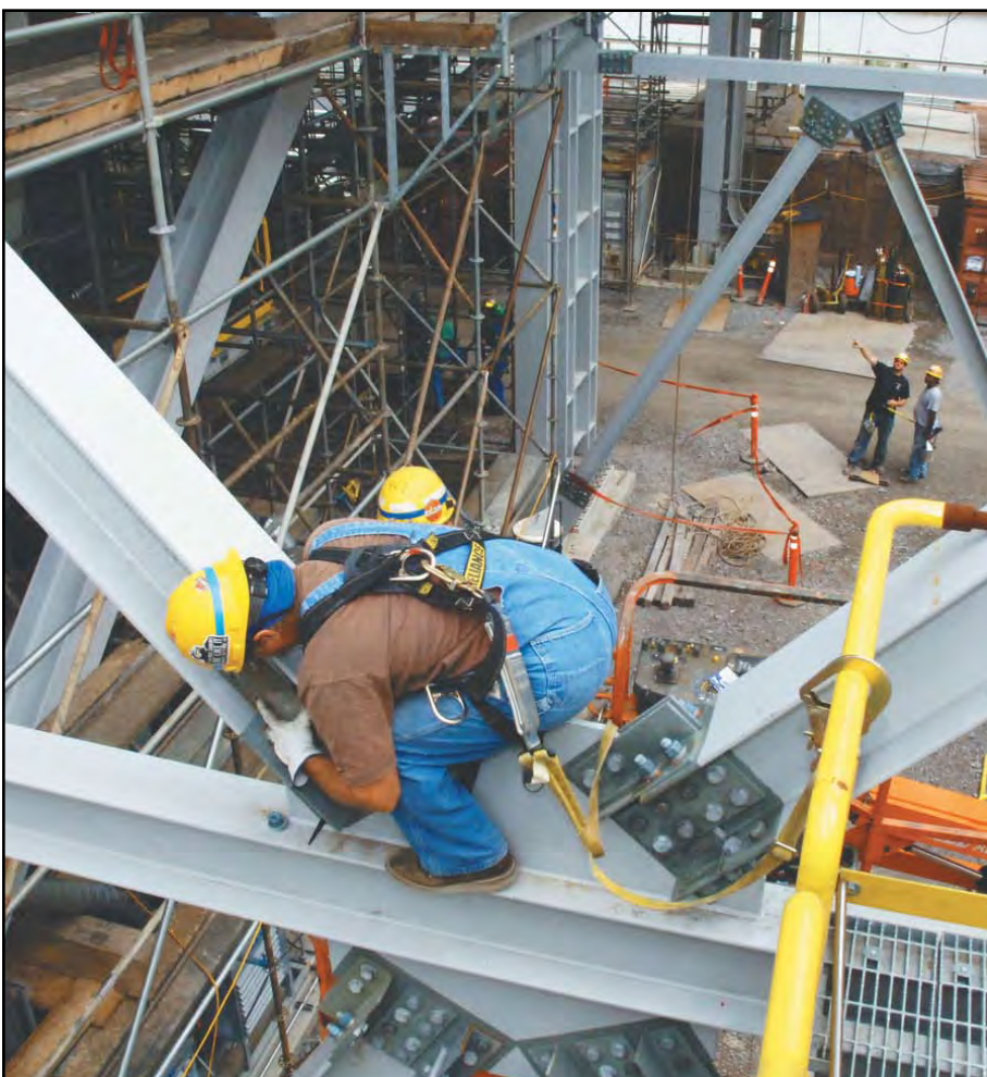
L-154 members detail breeching duct support steel at the W.H. Sammis Plant.
