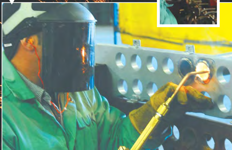
Luke Lafley, Local 242, removes a rolled tube using an oxygen-acetylene torch.
