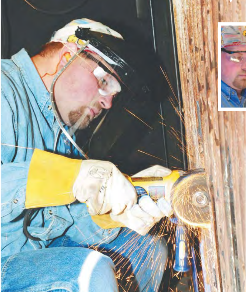
Ryan Woods, Local 27, grinds membrane during the water wall exercise.
