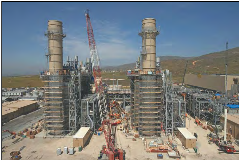
Local 92 members erect stacks in front of the HRSGs they are building at the new Otay Mesa Energy Center in Southern California.
