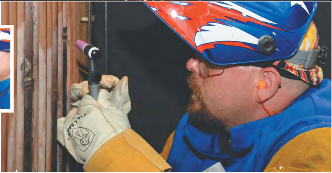
Eric Buskey makes a root pass using gas tungsten arc welding (GTAW) during the water wall exercise.
