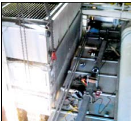
Local 28 members set one of three economizers into place at Princeton University in Princeton, N.J.
