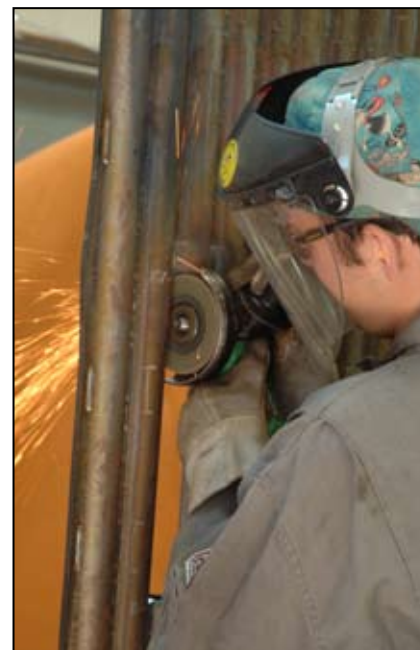
Dan Praught grinds waterwall membrane before fitting a replacement pup.
