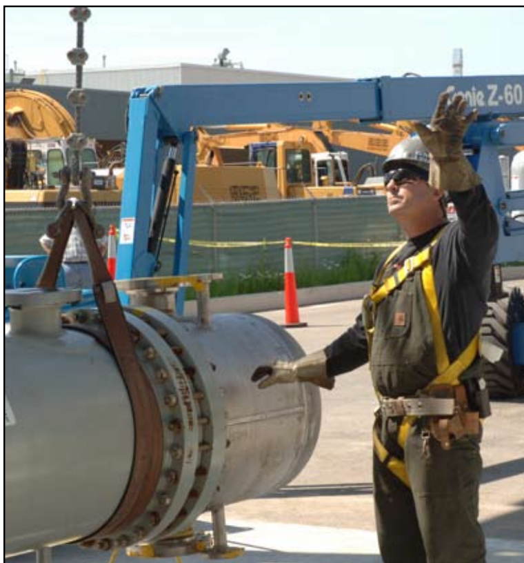
Greg Cameron, L-128, signals a tugger operator during the rigging exercise.
