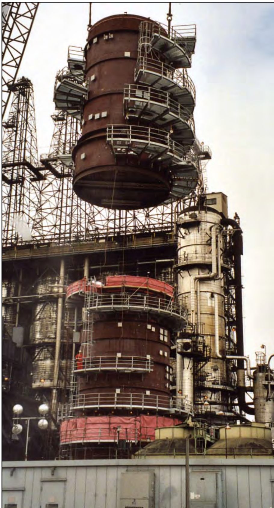
A shell section of a distillation tower (or fracturing tower) is set into place at the Chevron refinery in El Segundo, Calif., by L-92 members. Photos courtesy of Nooter Construction
