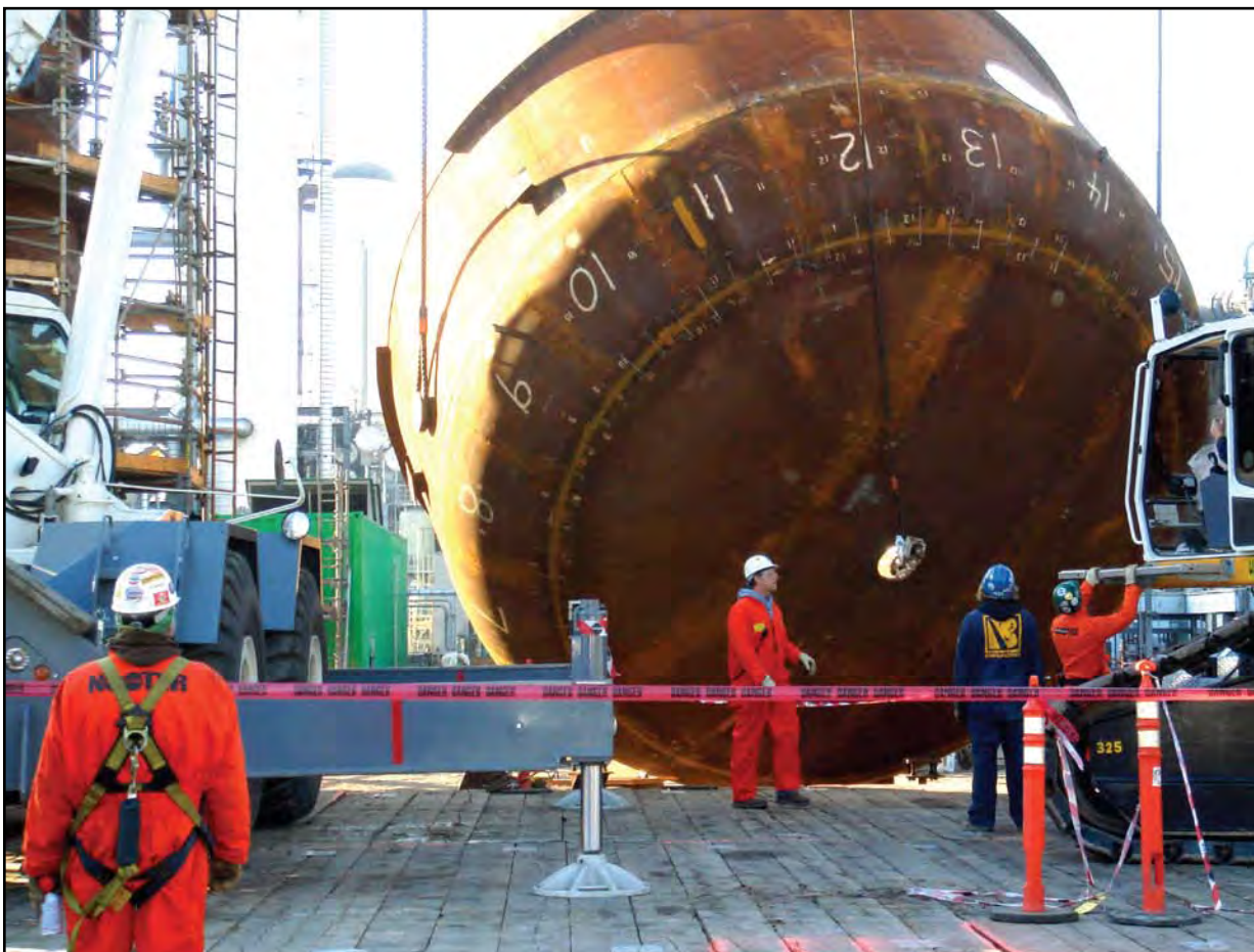
Local 92 members recheck the rigging on the bottom head of a fracturing tower before lifting it into place. Photo courtesy of Nooter Construction
