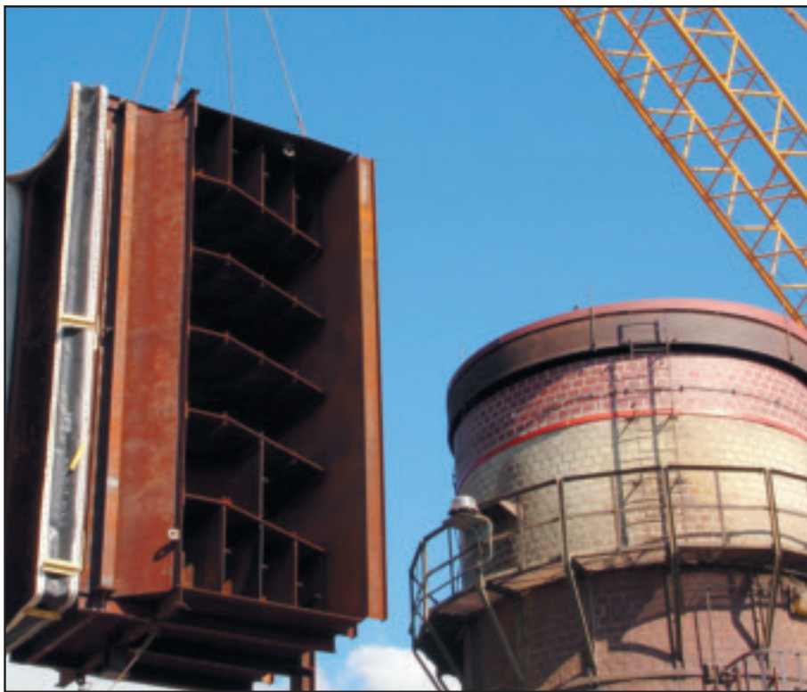
Local 193 members use a 365-ton crane to move a new ductwork section into place at the Mirant power plant on the Potomac River in Alexandria, Va. Sections ranged in size from 19,000 to 41,000 pounds.
