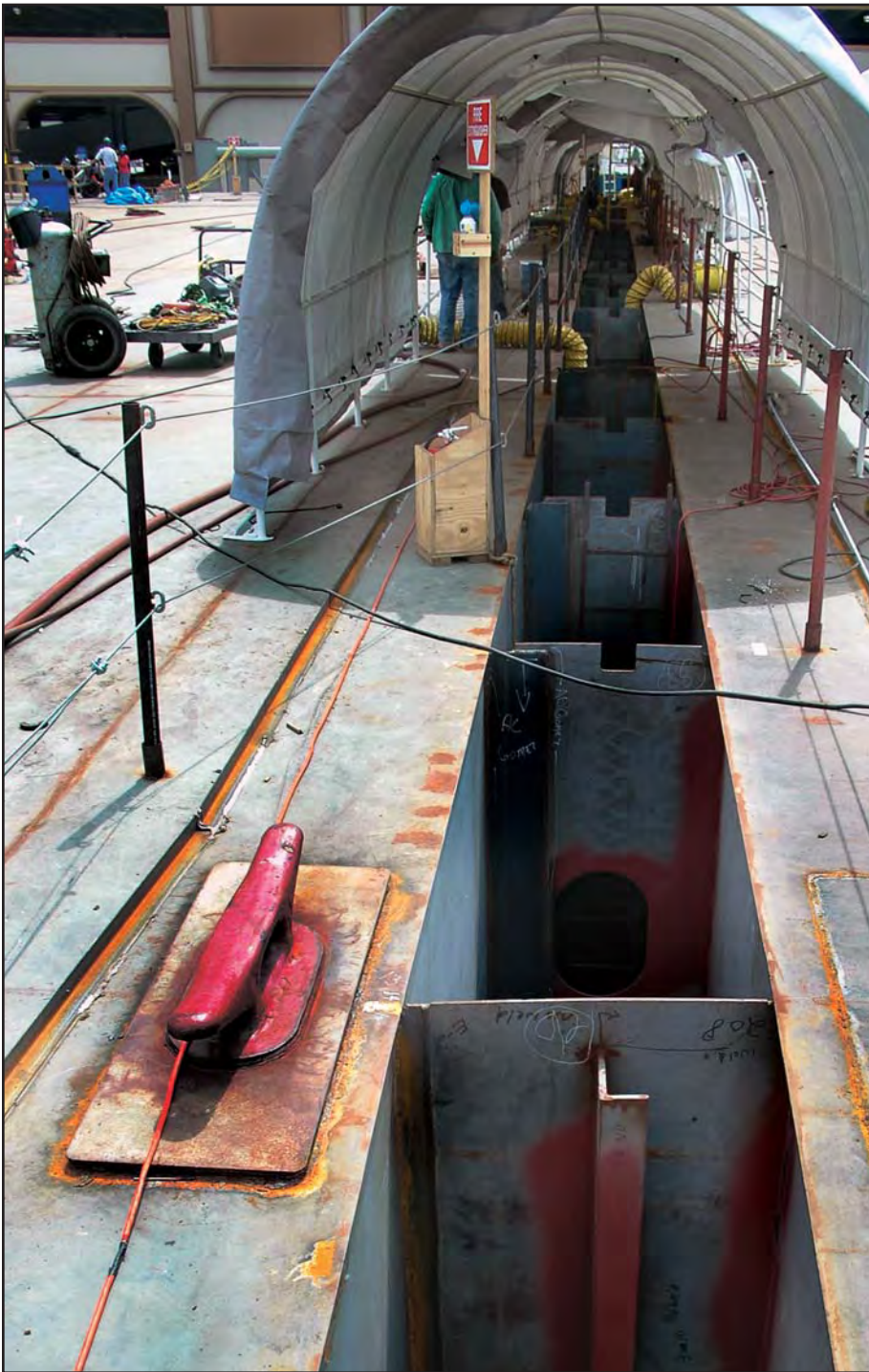
Local 374 members join two barges together. In all, they connected six barges to create the base for Harrah's new floating casino.
