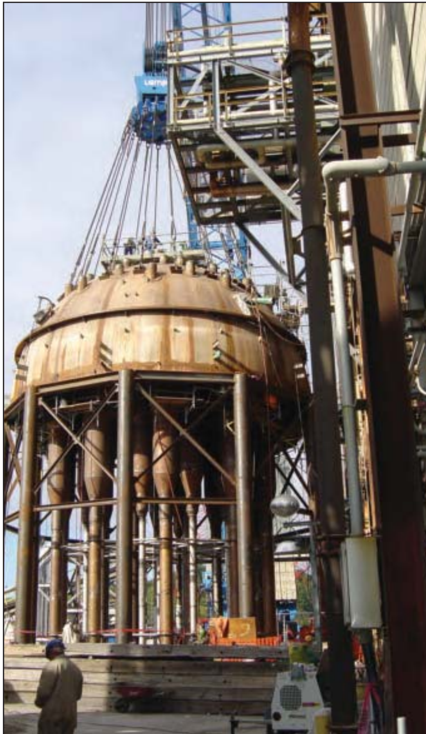
Boilermakers prepare to lift the rebuilt regenerator head in Catlettsburg, Ky.
