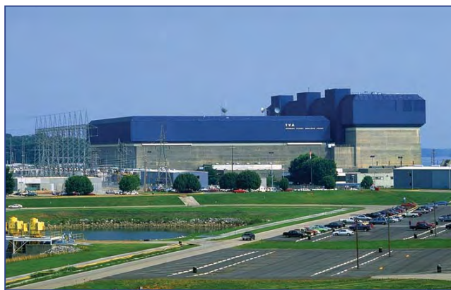
When Boilermakers completed the Browns Ferry Unit 1 in June, it became the nation's first nuclear unit to come online in the 21st century.
