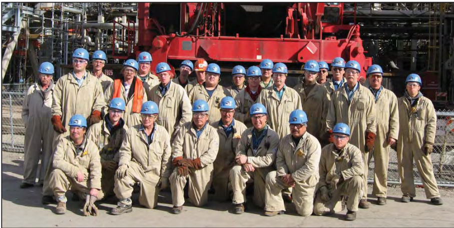
Local 11 Boilermakers are working the day shift at a plant-wide shutdown at the Conoco Phillips Refinery in Billings, Mont.
