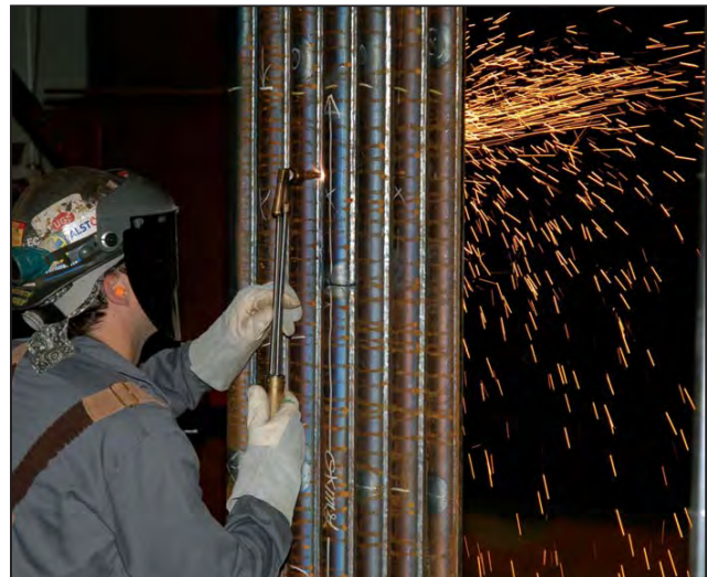
Martin Robichaud (L-271) cuts out the bad tube in the water wall exercise.
