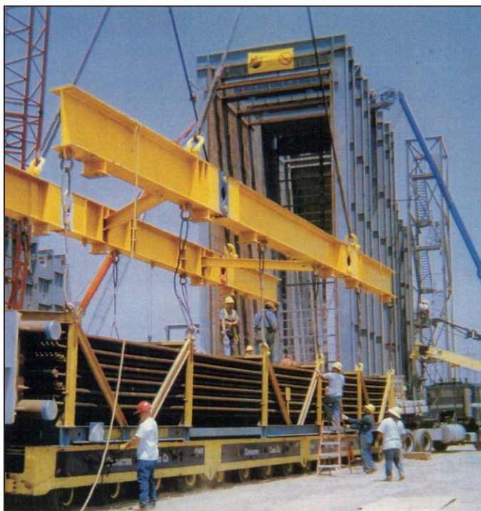
Members prepare to lift tube bundles during the construction project.
