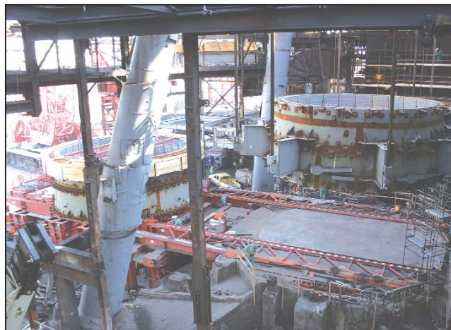
Local 374 members use strand jacks to raise new stack sections into place at Gary Works in Gary, Ind.
