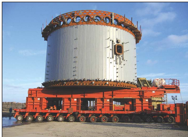
This multi-wheeled "Shirley car" is moving the new hearth for a blast furnace being built by Local 374 members.
