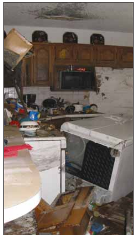
Although the outside didn't look too bad, when Joe entered his home he found nearly everything water-damaged beyond repair.
