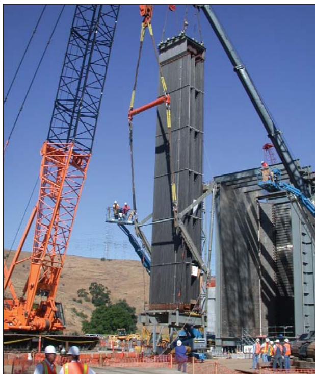
The first bundle goes into place at Calpine's San Jose HRSG installation.
