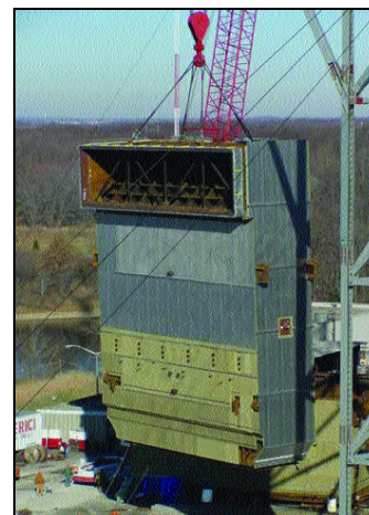
LOCAL 363 MEMBERS use "Big John" to lift ductwork measuring 65-feet high, 53-feet wide, and 14-feet deep.
