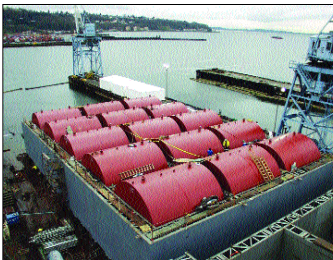
EACH OF THE CAISSONS being built by Local 104 members at Todd Pacific will be 130 feet by 80 feet by 225 feet deep.
