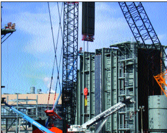
BOILERMAKERS FROM LOCALS 11 and 92 work hard for PSF Industries in Las Vegas, completing installation of two HRSG units eight weeks ahead of schedule.
