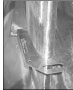
CLOSE-UP VIEW of square edges reprofiled by L-359 members to reduce & eliminate vibration and turbulence on a turbine.
