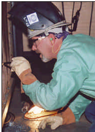
L-28'S JEFFREY HORTON representing the Northeast Area, inspects a tube cut as part of the welding/burning exercises.
