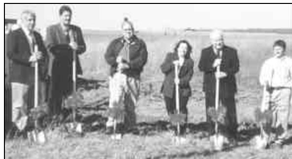
LOCAL 374 BREAKS GROUND for a new training facility in Dale, Ind. L to r., ABM Jerry Tempel, BM-ST Chuck Vanover, realtor Jerry Schue, Chamber of Commerce Pres. Becky Hochgesang, ABM Larry Seger, and instructor Jeff Schneider.
