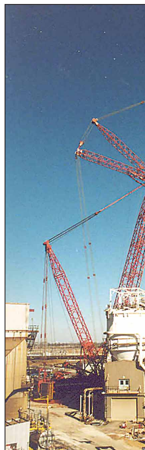
mobile crane, to set ductwork at a retrofit project for Ameren/CIPS.
