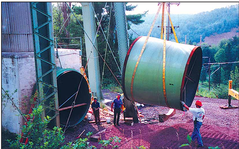
THE DAYS OF repairing leaks in the old wooden Victoria pipeline (at right) are history. Above, Local 169 members working for Azco Inc. install the first section of new pipeline below the surge tank at the bottom of the pipeline, above the Upper Peninsula Power Co.'s Victoria Hydroelectric Station.
