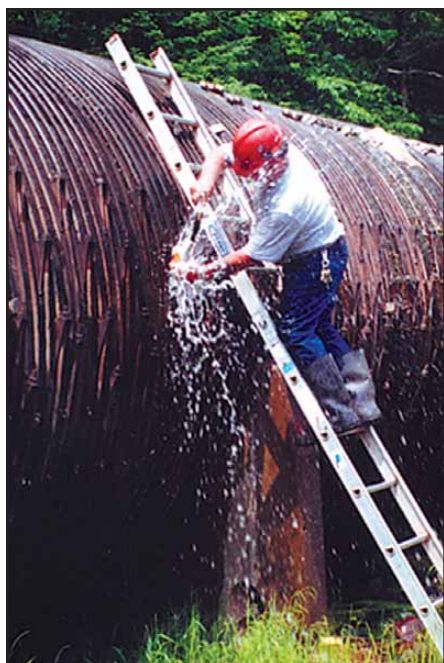
THE DAYS OF repairing leaks in the old wooden Victoria pipeline (at right) are history. Above, Local 169 members working for Azco Inc. install the first section of new pipeline below the surge tank at the bottom of the pipeline, above the Upper Peninsula Power Co.'s Victoria Hydroelectric Station.
