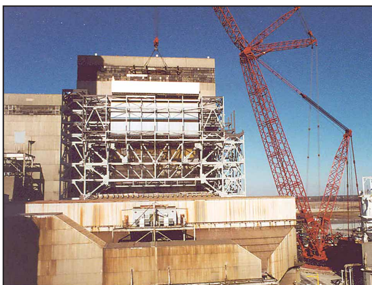
mobile crane, to set ductwork at a retrofit project for Ameren/CIPS.
