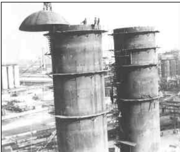
IN THE 1960S, LOCAL 359 members place a top on a digester in Prince George.
