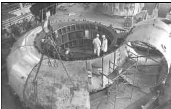
IN THE 1970S, LOCAL 359 members assemble the first scroll casing in a Vancouver shop, following its arrival from Japan for the Mica Creek dam in British Columbia.
