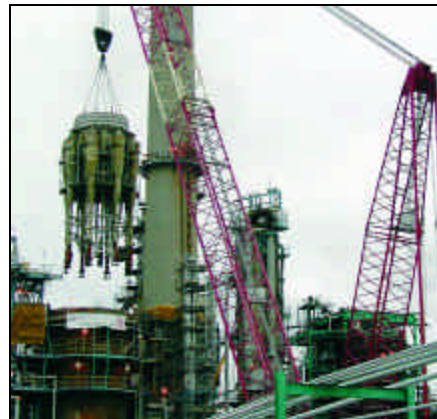
PART OF THE FALL turnaround at the Imperial Oil Refinery in Samia included installation of a 135-ton cyclone/plenum.
