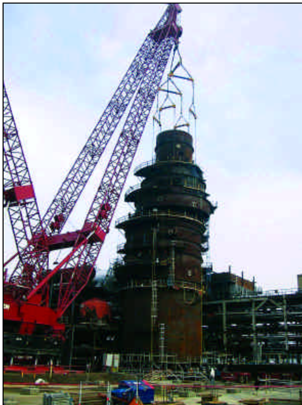
HERE'S ANOTHER VIEW of the lift for the vacuum tower assembly. Local 146 members use a PTC 2000 metric ton crane to lift the 430 short ton unit.
