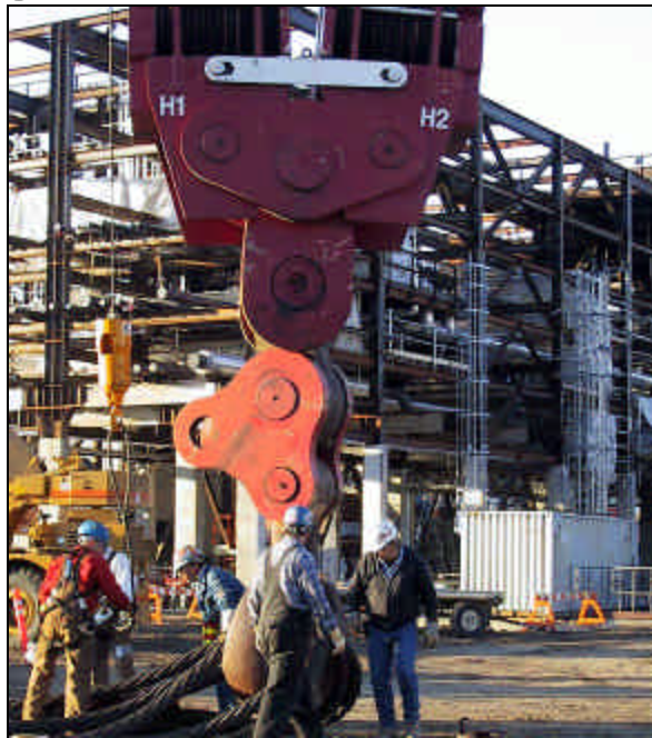
LOCAL 146 MEMBERS RIG a PTC 2000 metric ton crane hook (block weight 75,000 lbs.) to lift a vacuum tower at the Shell Scotsford upgrade.
