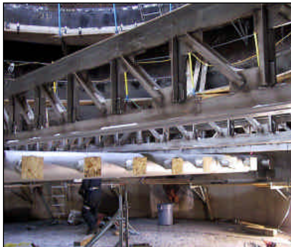
MEMBERS OF LOCAL 146 install the internal trusses of a vacuum tower during an upgrade/expansion project for the Athabasca Oil Sands Downstream Project.
