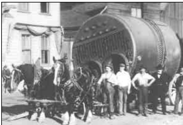
IN 1892, WORKERS USE horses to deliver this scotch marine boiler for the S.S. Joan built by Boilermakers at the Albion Iron Works in Victoria, British Columbia.
