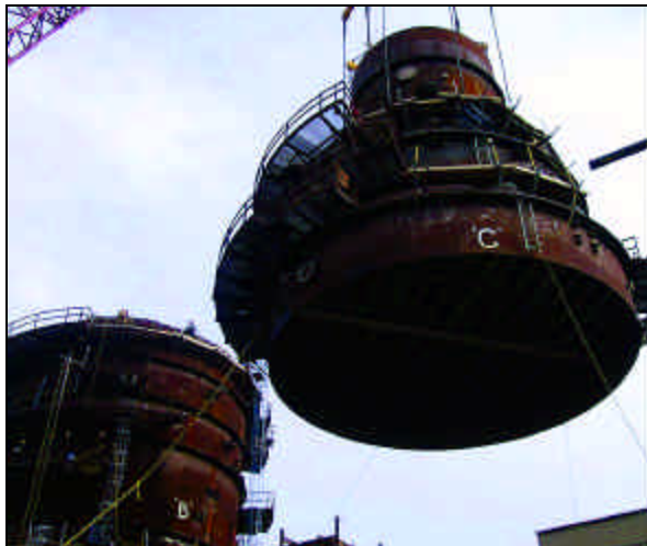
MEMBERS OF LOCAL 146, Edmonton, Alberta, Canada, lift the third assembly of the vacuum tower during an upgrade/expansion project.
