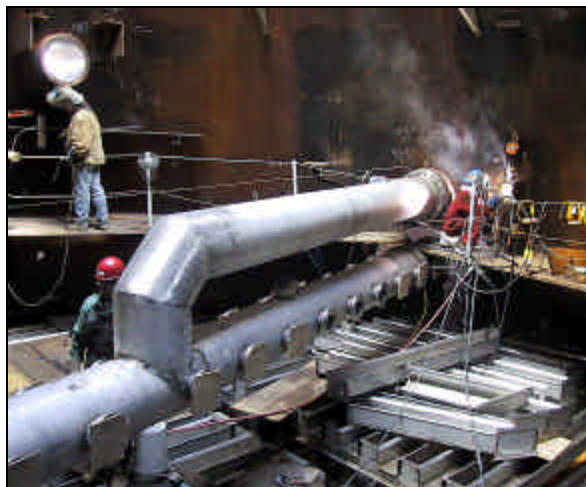
AFTER THE VACUUM TOWER is assembled, Local 146 members begin the internal work.
