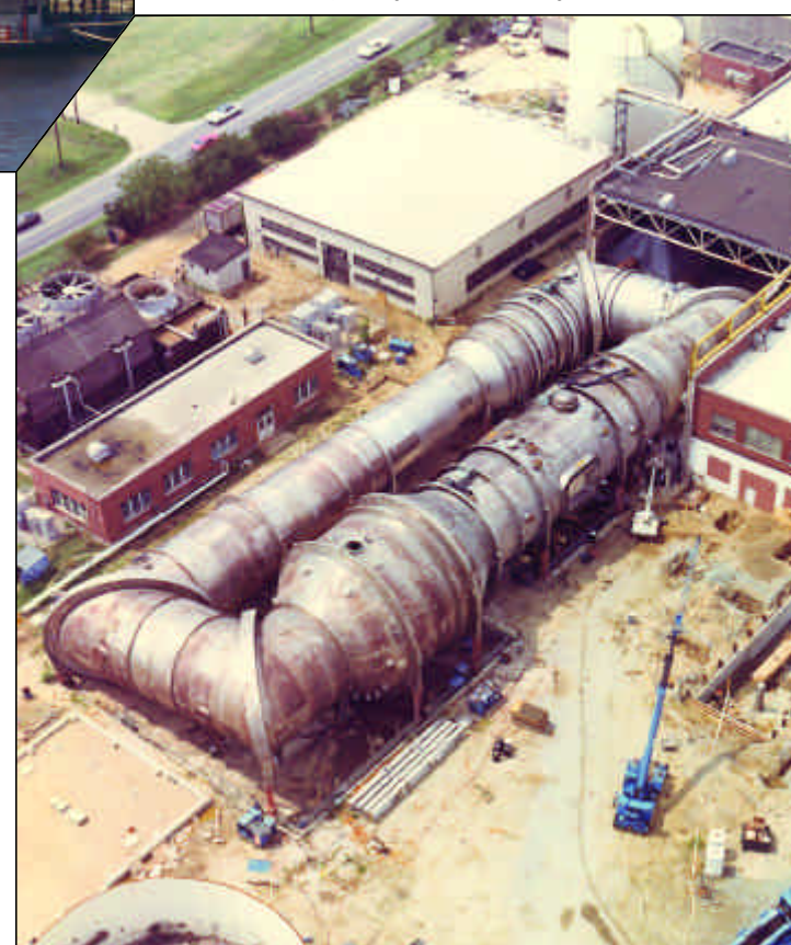
MEMBERS OF THE NTL joined Local 92 members of Los Angeles, Calif., working for CBI, to build this wind tunnel for Boeing Aircraft at Moffet Field, Calif.
