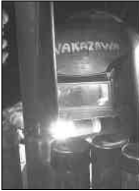
TIG welder Brian Nakazawa replaces 30-year-old tubes in a tight-wall boiler.
