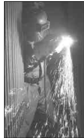
Lloyd Moores uses a carbon arc torch to gouge a tube wall.
