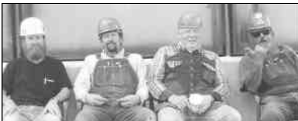
Building tanks for the Morse Construction Group, are, l. to r., foreman Ray Peit of Local 502, Tacoma, Wash.; Dick Lockyer and asst. foreman Ron "Skip" Holt of Local 182, Salt Lake City, Utah; and Cliff Aken of Local 204, Honolulu, Hawaii.
