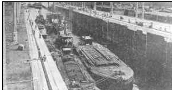
In 1913, these ships await the first lockage from sea level up into Lake Gatun, a surface elevation of 85 feet above sea level.
