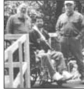
L-83 members R. D. Downs (left) and Rick Delay (right) built this ramp and deck for injured member Mark Suthers.
