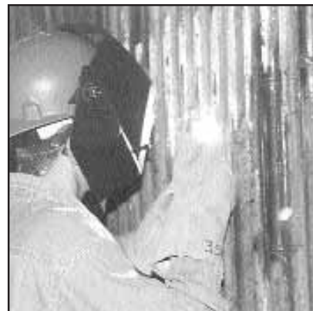
Jason Verge of Local 28, representing the Northeast Area, at left, buddy welds a tube with Robert Hummel of Local 7.
