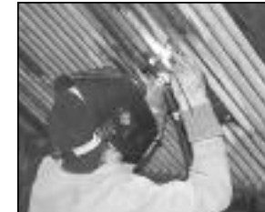
Paul Hendershot of L-7, Buffalo, N.Y., replaces a tube section in a water-wall panel during the welding competition.
