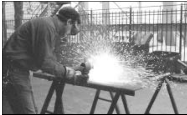
BNAP Instructor John Standish demonstrates how to use a thermal sprayer. Prime Alloys of Houston, Texas, and Boyd Machine & Repair of Wolf Lake, Ind., loaned the Mark II Twin-Wire Arc System to the Boilermakers National Apprentice Program (BNAP) for a six-month period at the national training center in Kansas City.
