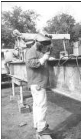
L-154's Harris prepares to weld lifting lugs.
