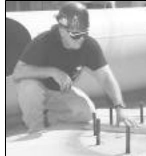
Terry Weaver (L-374) measures an area where he must place a glass-lined vessel during the rigging exercise.
