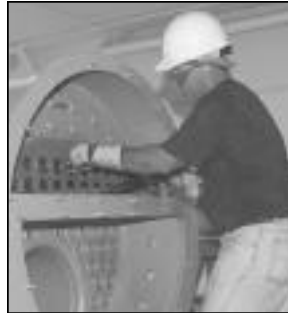
Second-place winner Robert Dolce (Local 7) performs tube-rolling as part of the hands-on skills testing.
