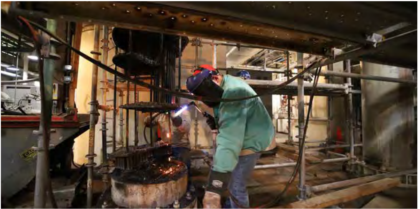
Workers remove old tubes in preparation for a potential biomass conversion in one of the plant's boilers.
