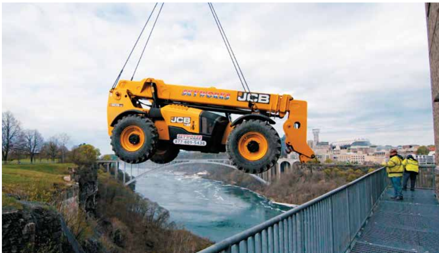
Boilermakers fly equipment down the 200-foot gorge in preparation for building the new vessels.
