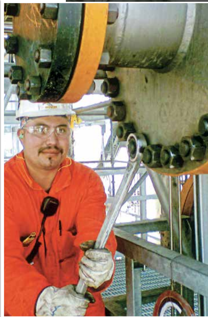
In 2006, Oscar Davila works as a foreman for Nooter Construction at the Valero Wilmington Refinery. Here he’s blinding a vessel for testing.
