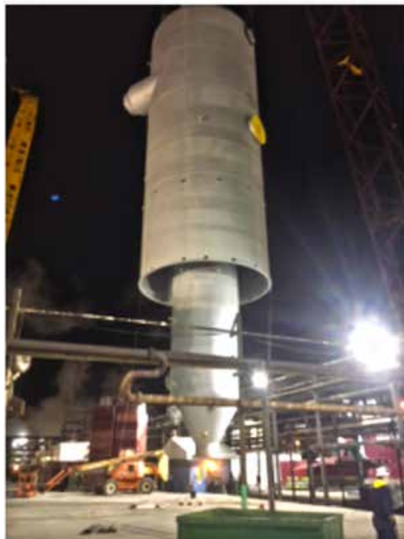
Boilermakers working for Madison Industrial lift the new reactor into place.
