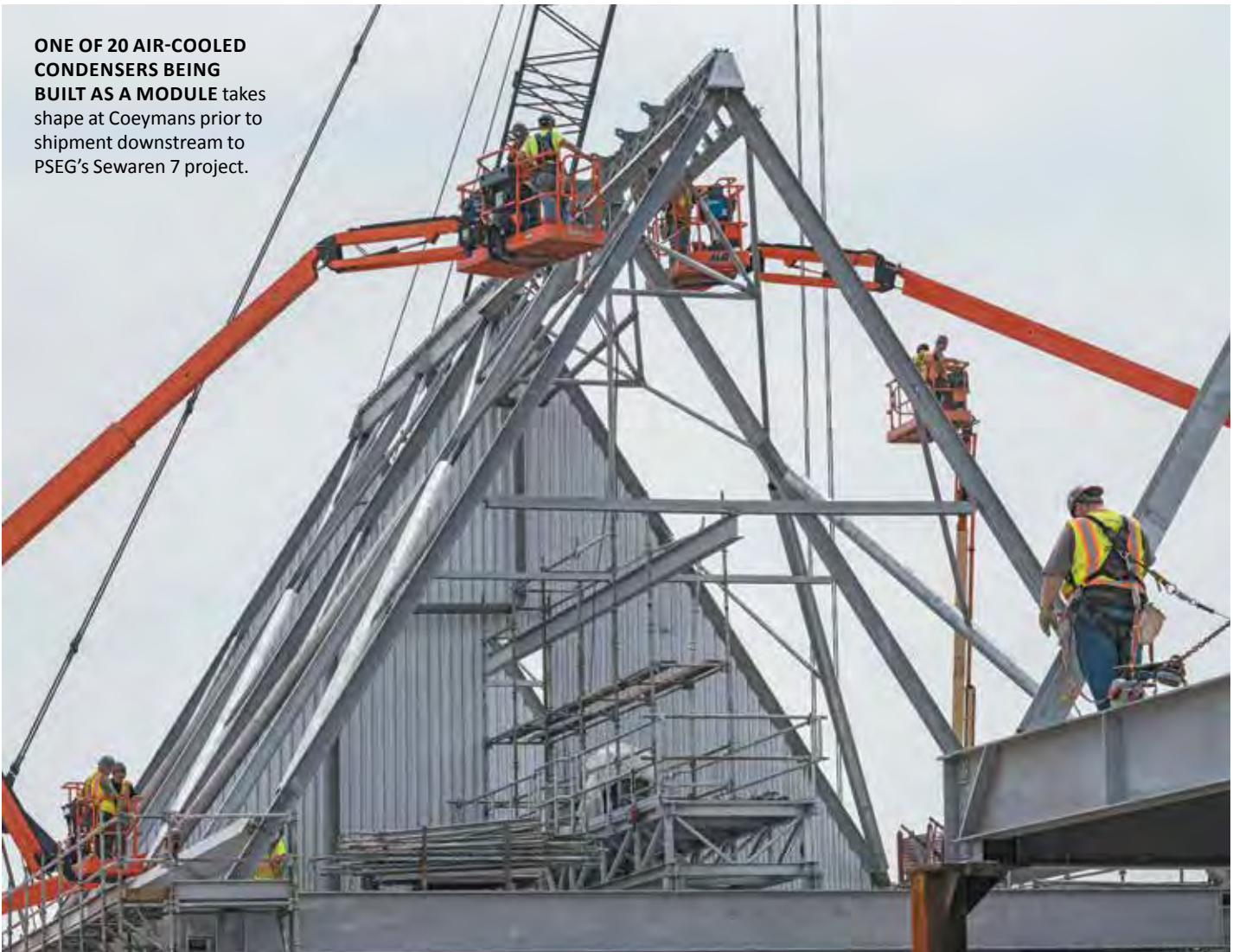
TRAVELING BOILERMAKER BILL HERNDON, LOCAL 27 (St. Louis) , welds set-up material for one of 20 air-cooled-condensers.
