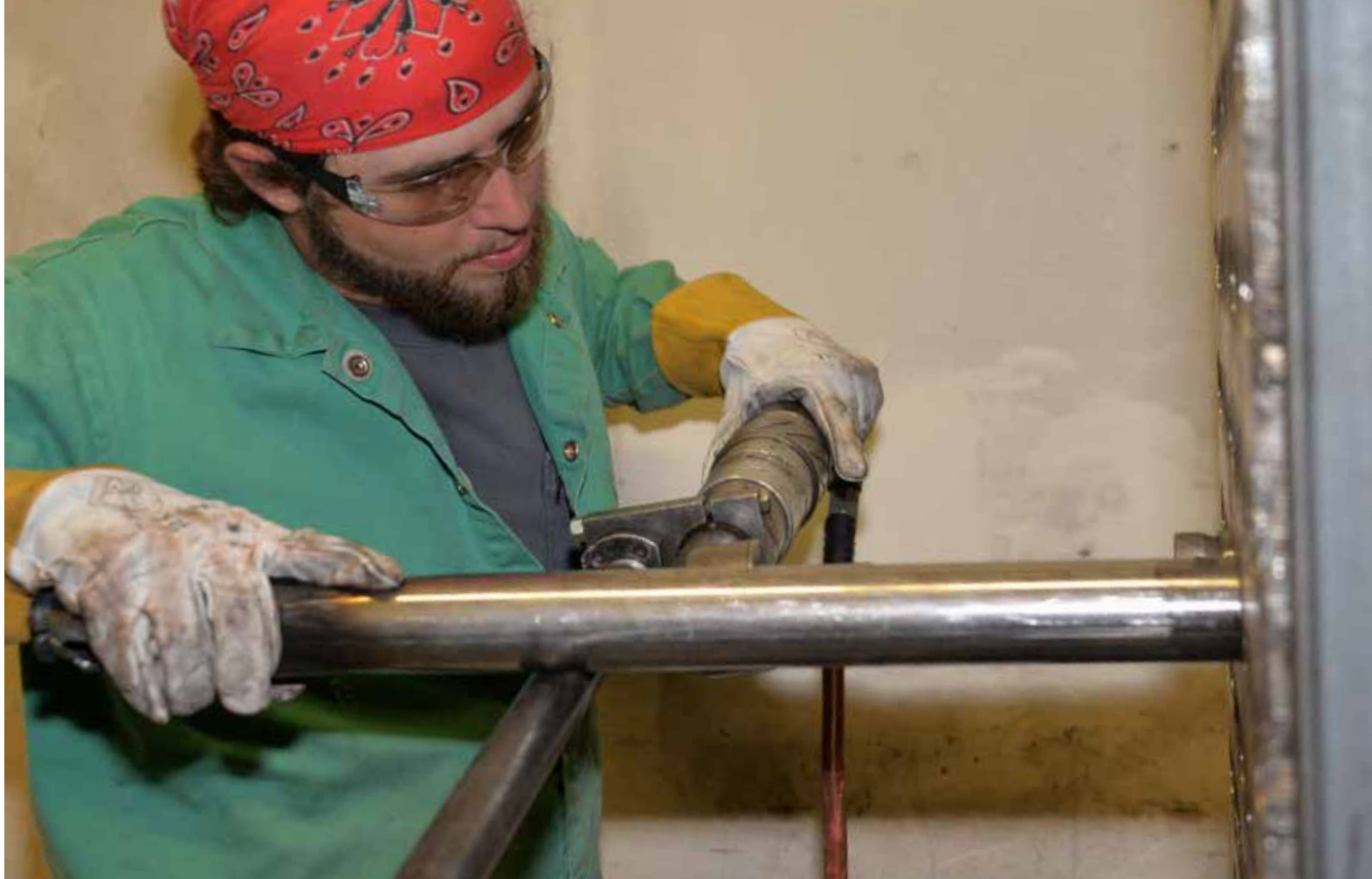
CHANCE ELLISON, L-108, PREPARES TO REMOVE THE FINAL INCHES OF TUBE STOCK DURING THE TUBE ROLLING PROJECT. ▲
