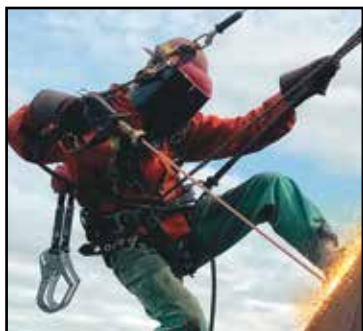
LOCAL 169 APPRENTICE JUSTIN ZUESKI lances (cuts apart) a downcomer at U.S. Steel's River Rouge plant near Detroit in May 2017. Photo courtesy J. Williamson.
