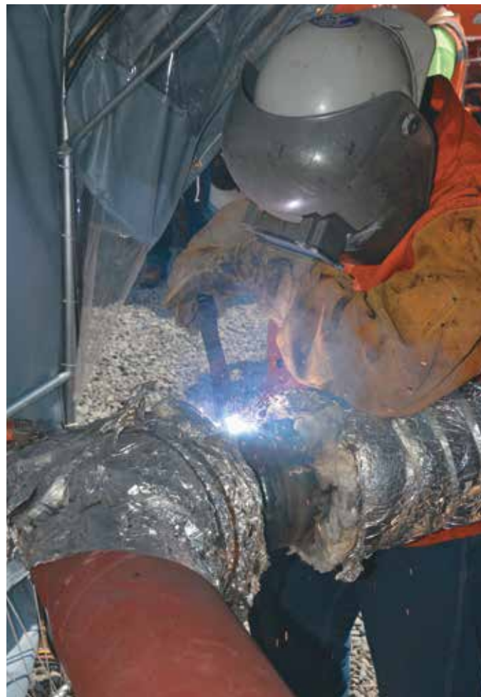
MIKE CRUGNALE, L-13 , welds a downcomer, which will carry cold water from the steam drum as steam is condensed and recirculated.
