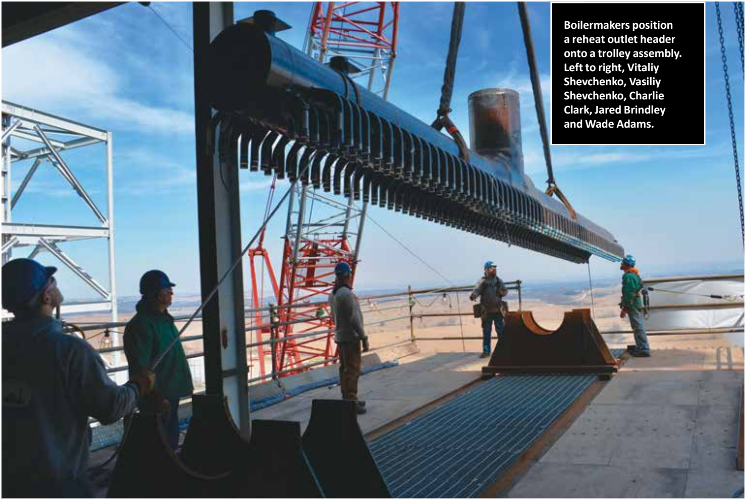
Crew members disconnect rigging following a successful lift to the penthouse platform.
