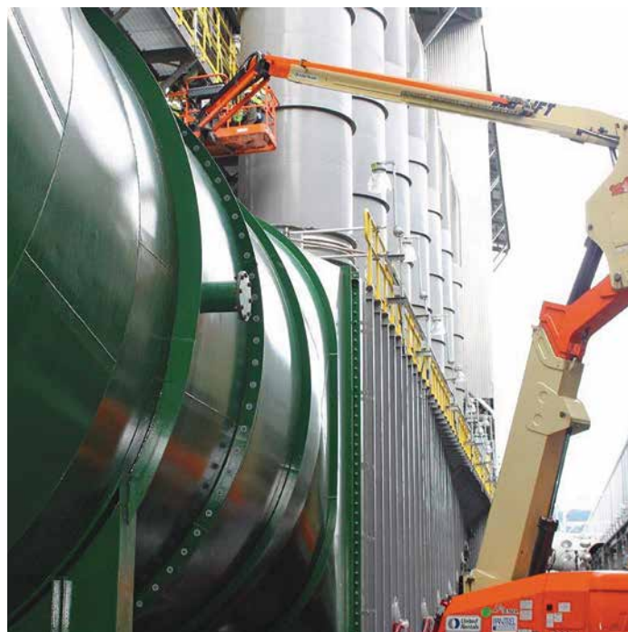
PART OF THE TWO KILOMETERS of ductwork installed by Boilermakers.
